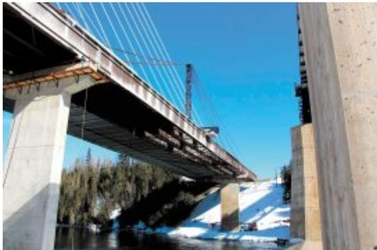
Instead of demolishing the old Nipigon River bridge, engineers offered a more efficient option by rolling the bridge across its piers and then gradually dismantling it on shore. - Photo: Andrew Van Gilst
